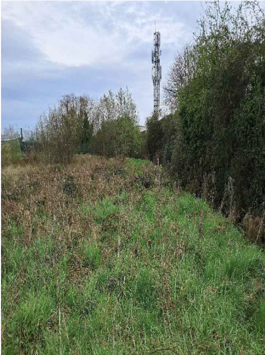
Mast at Train Station
